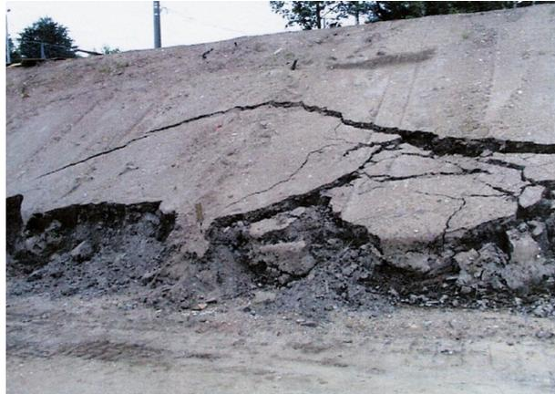
Fig. 62 shows the embankment slide due to faults in the slope toe.
